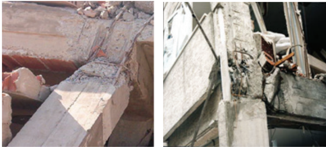
Fig 1. Failure of Beam-Column Joint
