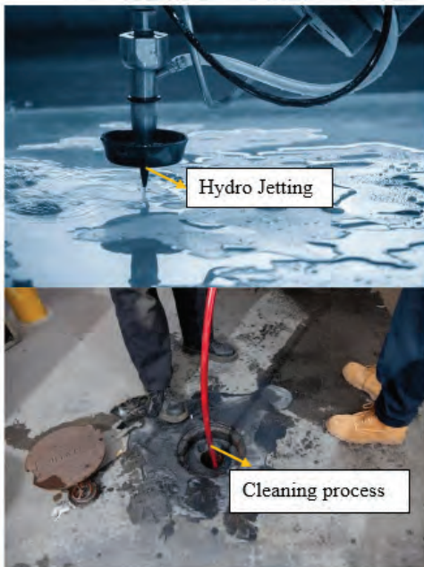
Fig. 2 Hydro Jetting Method
