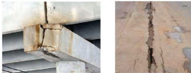
Fig. 2 Fatigue crack on (a) structural component (b) bridge deck pavement (Suryavanshi 2010)
