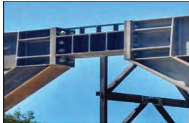
Fig. 2. Eccentric braced frame
