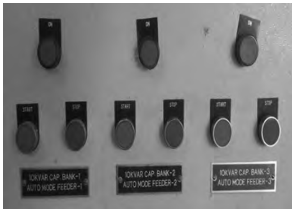
Fig. 9 Reactive load of 30 KVAR
