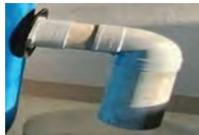
Fig. 10. Kitchen waste inlet pipe
