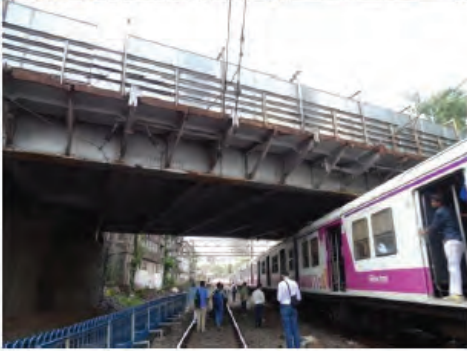
Fig.1. Actual site photo of the existing skew bridge located in Mumbai, India
