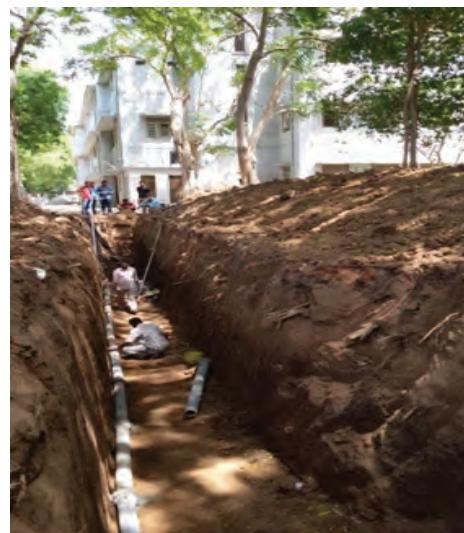
Fig 4: Experimental setup of Horizontal BTHE
